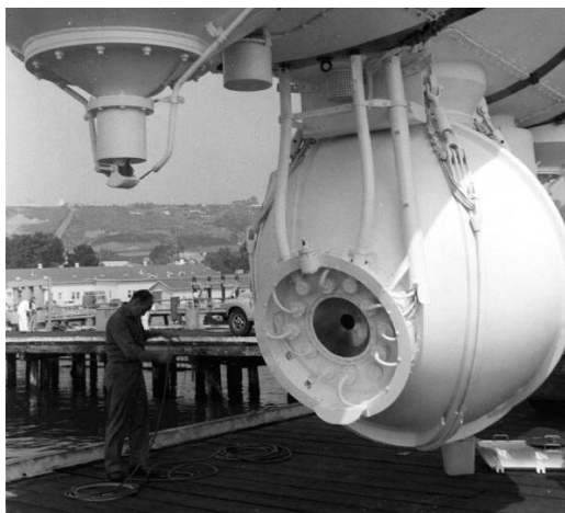
Photo # NH 96805 Trieste's pressure sphere, ca. 1958-59
